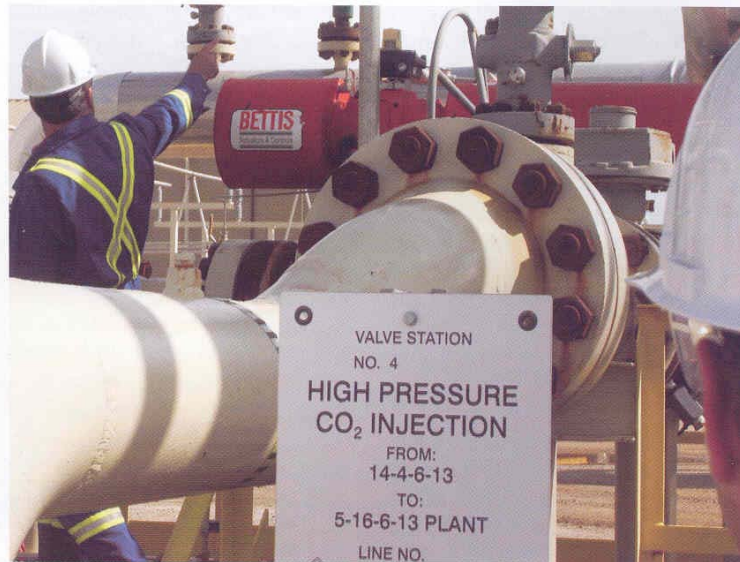
The CO 2 Pipeline Close-up. More than seven million tonnes of CO 2 captured from the Dakota Gasification Plant in Beulah, North Dakota has been transported 320 km via pipeline to the Weyburn field, where it is now securely stored 1500 metres underground in depleted oil and gas reservoirs.
